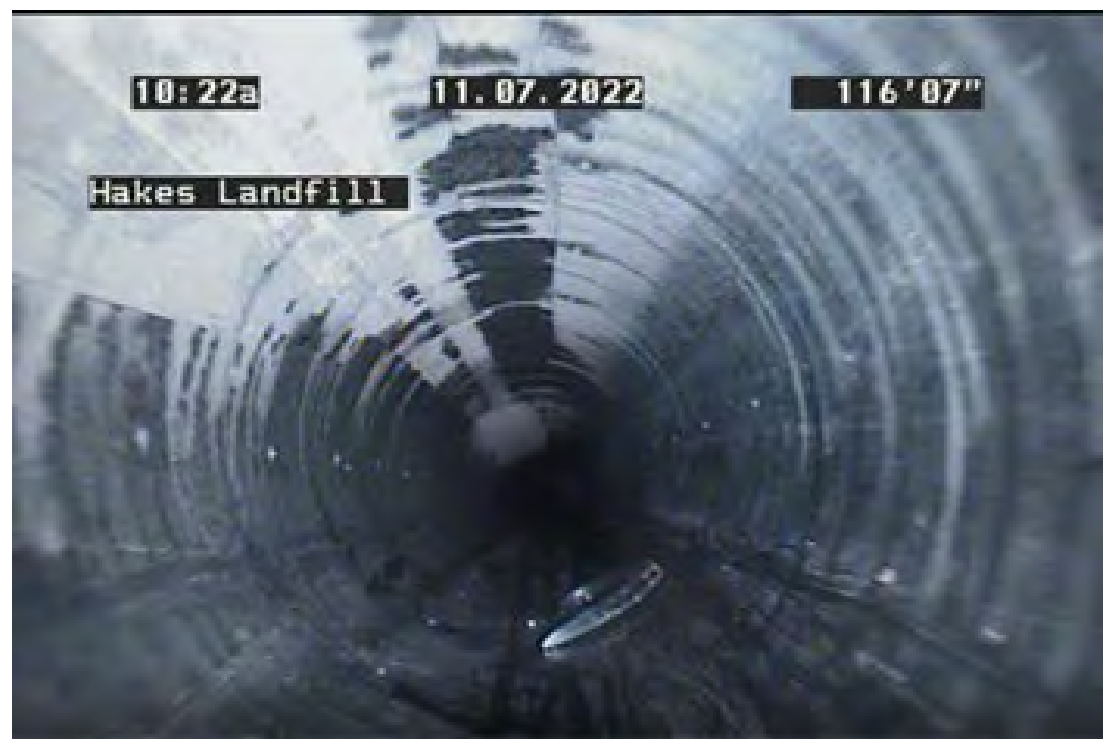
Photo showing strip of HDPE from debeading activities
