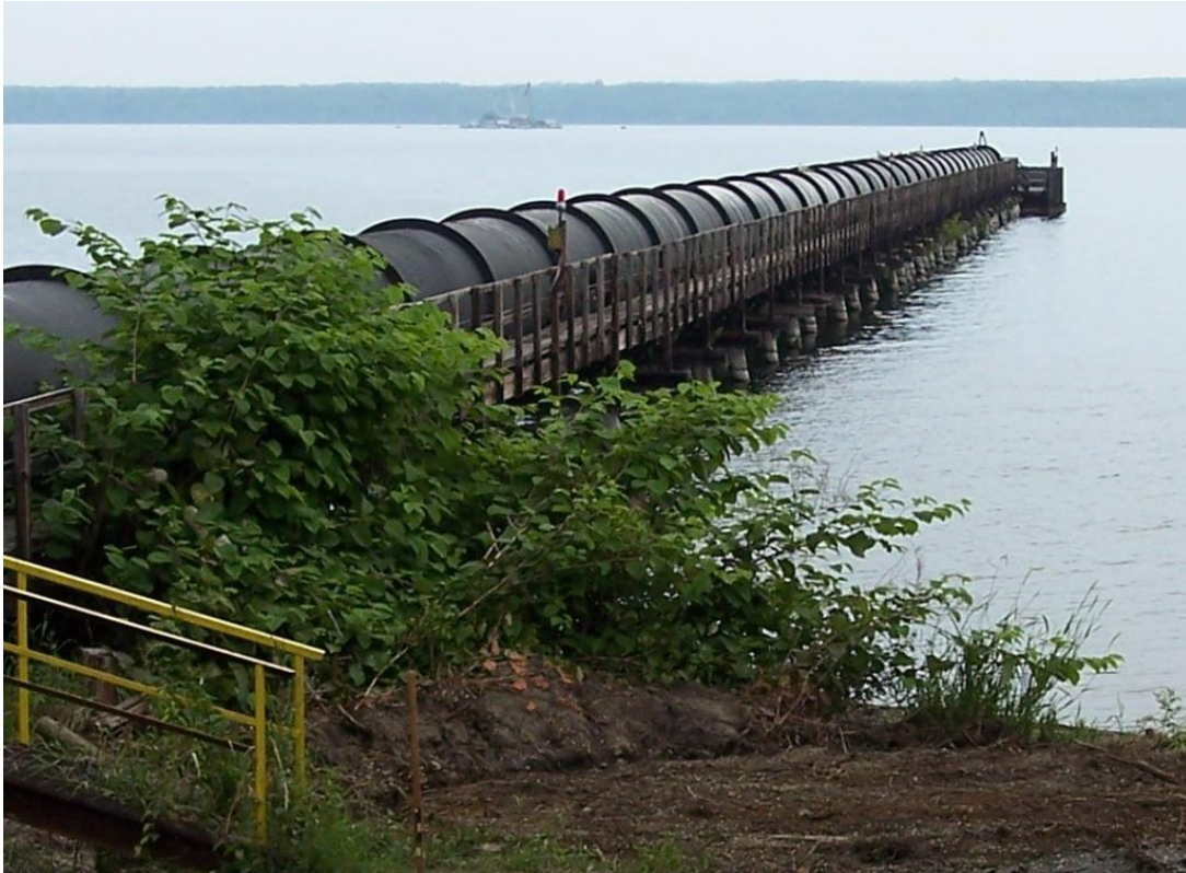
Figure 2-2 Unit 4 withdraws water from an elevated 7-ft diameter conduit that extends 650 ft from the west shore of Seneca Lake, and 1900 ft from the pumphouse.
