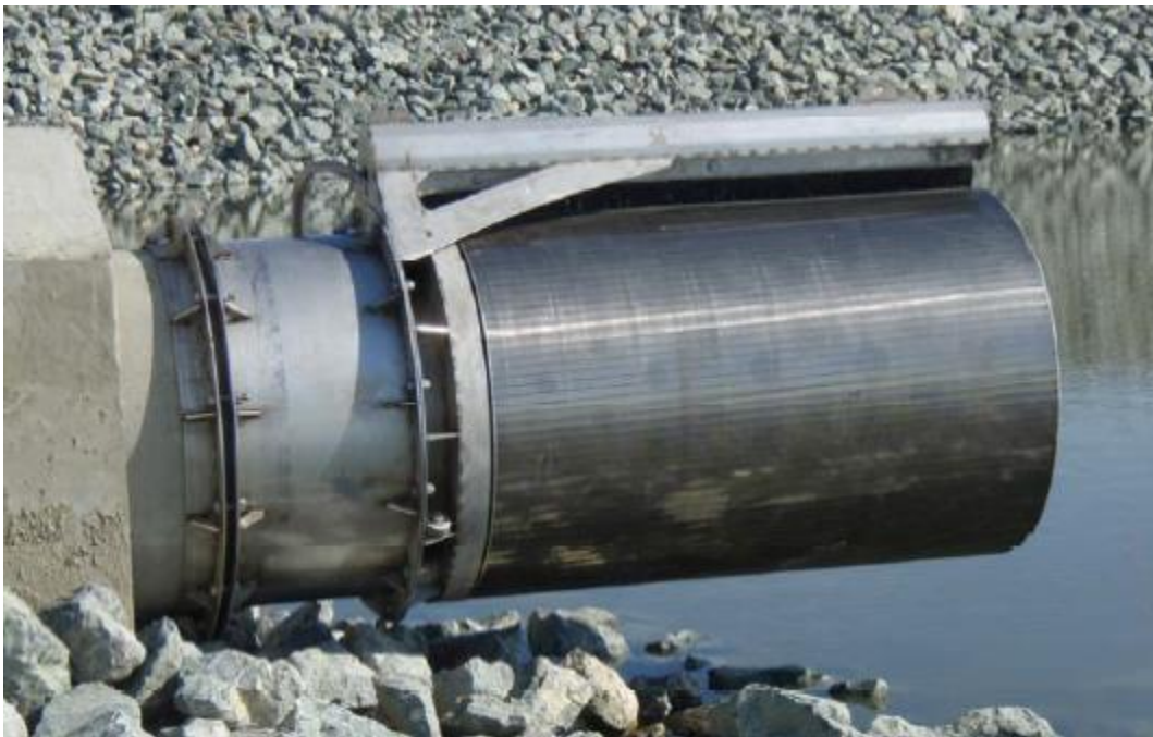
Figure 3-2 Example of horizontally mounted cylindrical wedgewire screen with external cleaning brushes.
