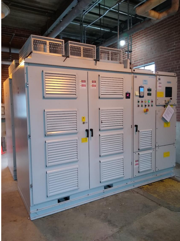
Figure 4-2 Variable frequency drive units installed in the GGF pumphouse.
