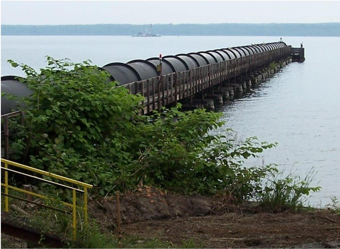
Figure 2-1 Unit 4 withdraws water from an elevated 7-ft diameter conduit that extends 650 from the west shore of Seneca Lake.
